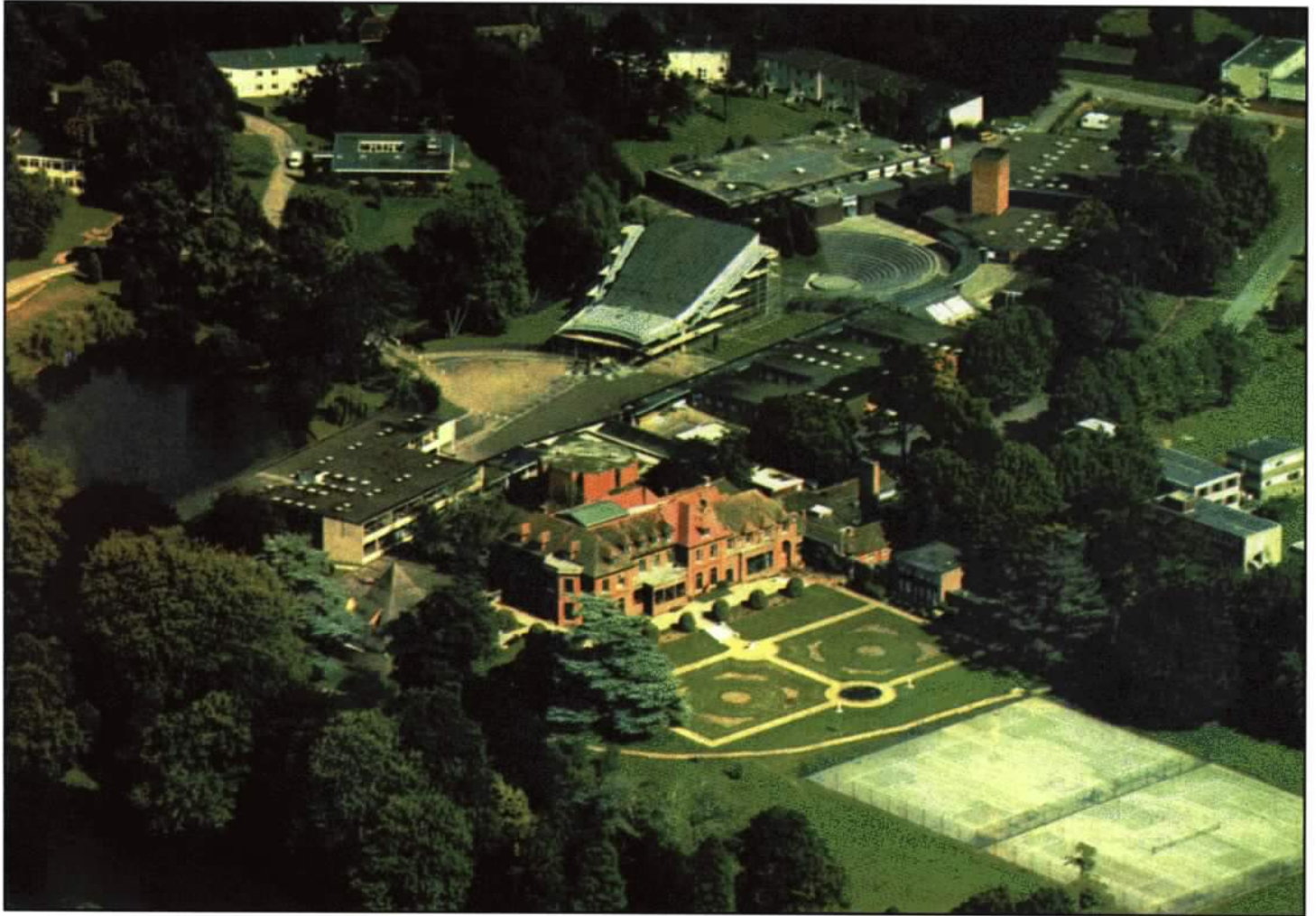
Aerial view of the Carmel College site at Wallingford near Oxford.●
